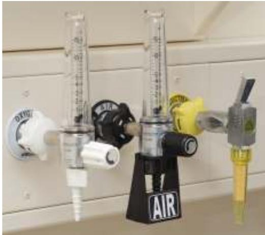
*Fig. 1: Air clearly different to oxygen*
